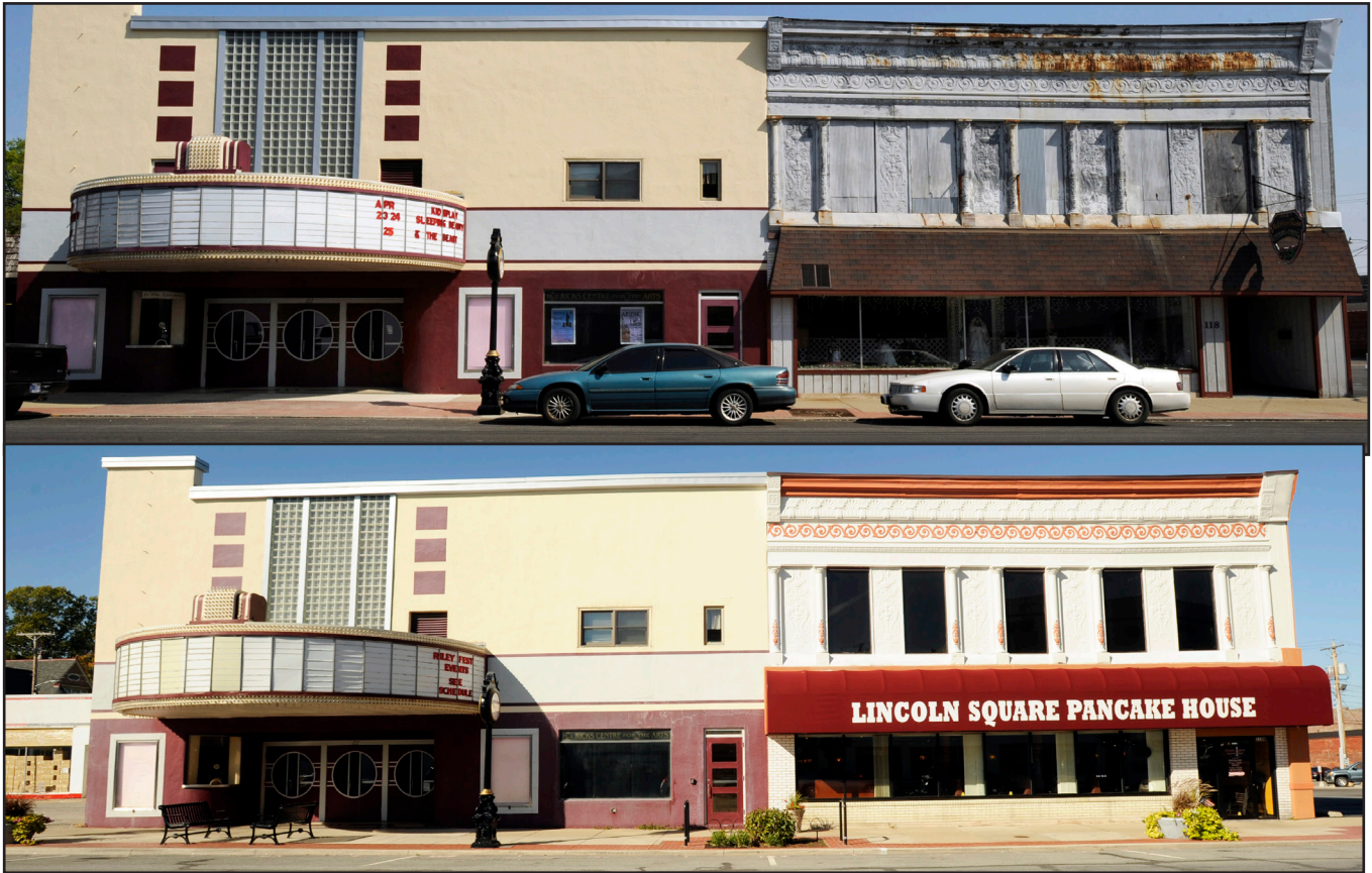
Before (top) and after (bottom) images of a revitalization project within the downtown.
