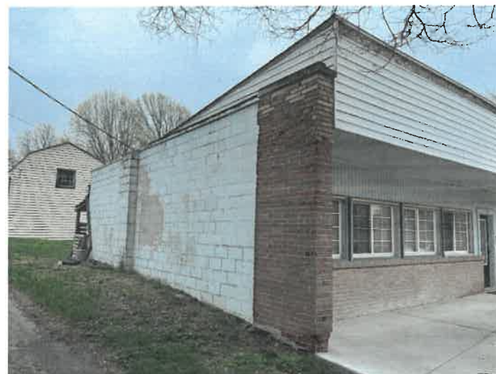
Existing Northwest Corner
