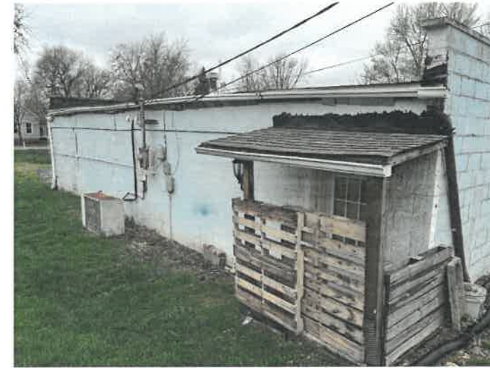
Existing Northeast Corner
