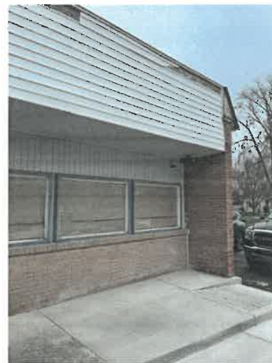
Existing Southwest Corner
