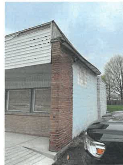
Existing Southwest Corner
